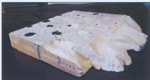
Picture 4: PU specimen removed from the flat roof
