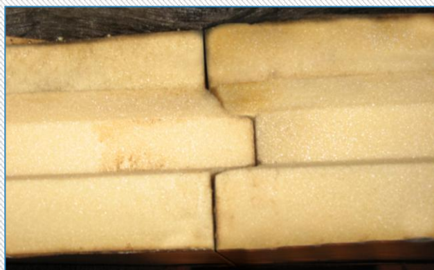
Picture 3: Insulation boards tightly installed against one another
