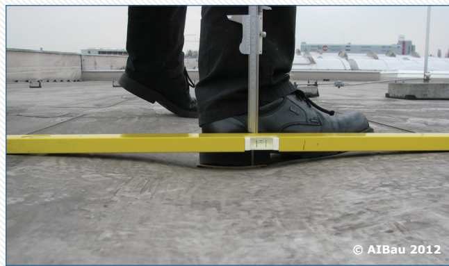
Figure 5: Measurement of the deformation [1]
