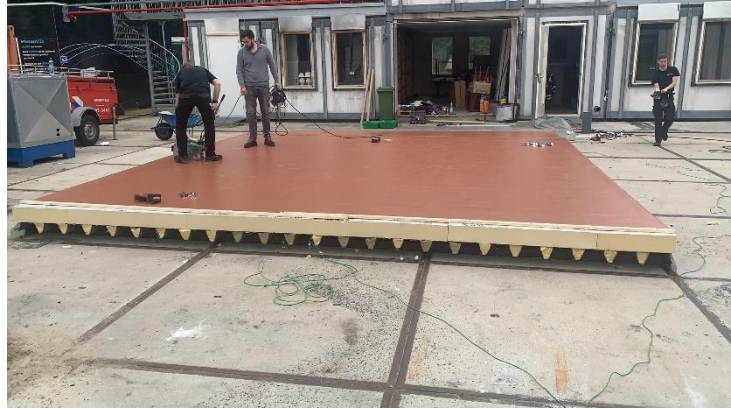
Photo 23 The roof waterproofing sheet is welded.
