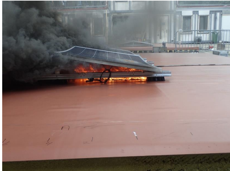
Photo 8 The fire is spreading underneath the PV modules (time 10:13).
