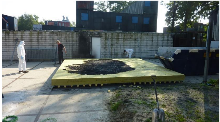
Photo 15 Overview of the burnt section of the MW insulation (top layer).
