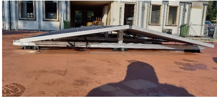
Photo 24 The PV modules have been positioned.
