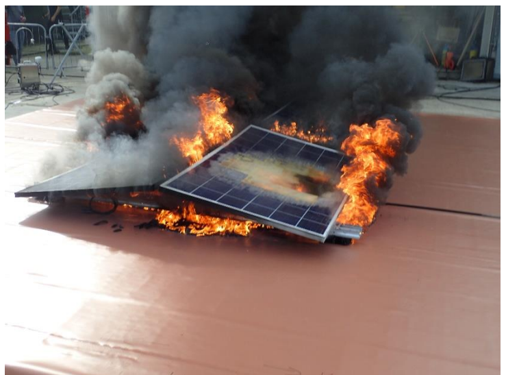
Photo 28 The fire is spreading underneath the PV modules (time 15:06).
