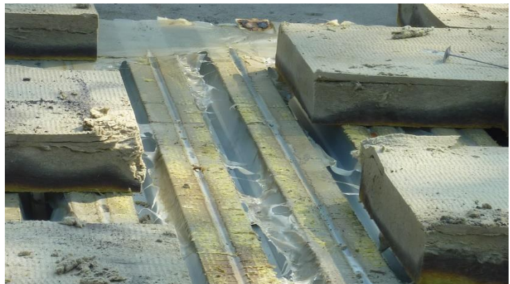
Photo 19 Detail of the burned vapour barrier.
