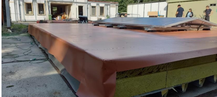
Photo 4 The PV modules have been positioned.
