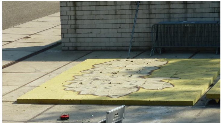
Photo 17 Overview of the burnt section of the MW insulation (underside of top layer).
