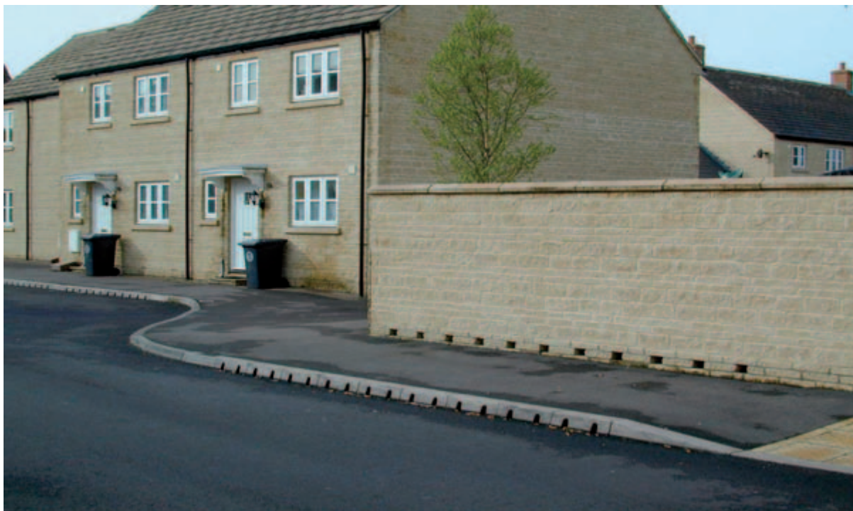
Figure 5.1 Drainage relief openings (courtesy of HR Wallingford Ltd.)
