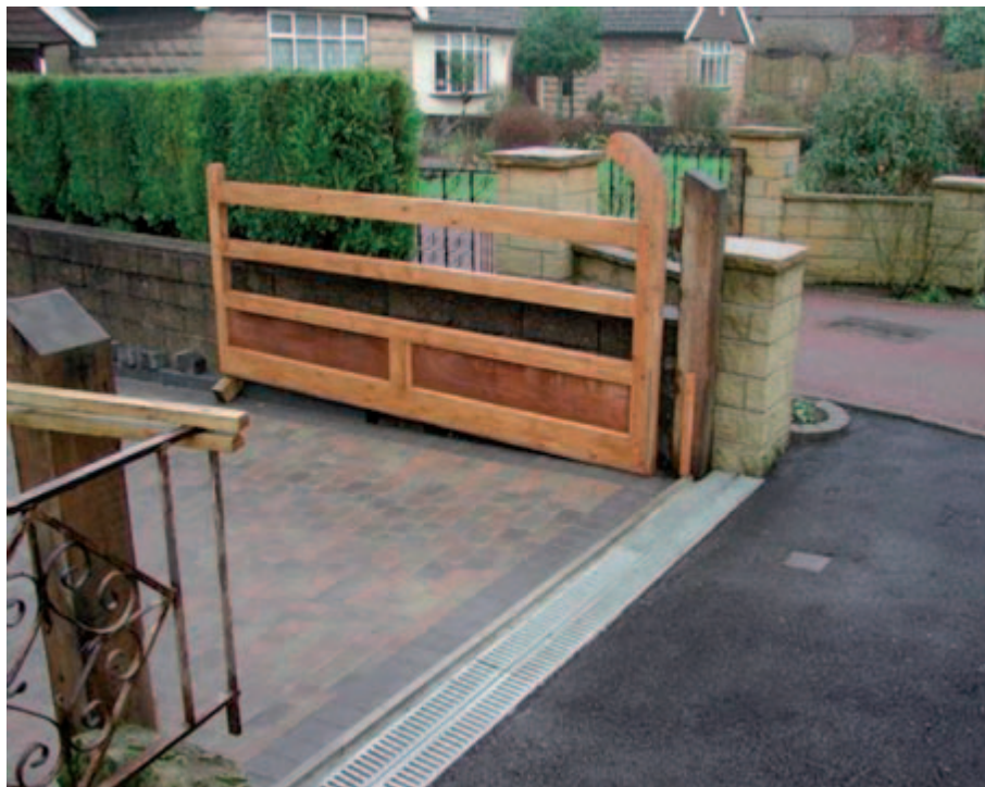
Figure 5.4 Example of property boundary wall and lower sealed gate (courtesy of Severn Trent Water)
