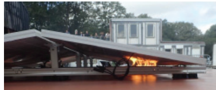
Figure 1: PV array on the flat roof after ignition of the gas burner
